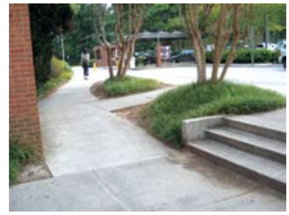
Fig 7: All change in levels should be negotiated by ramp, this is helpful for all children
